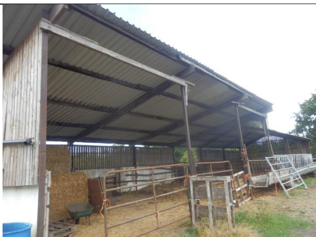
Photograph 23: Open-sided farm building with wooden cladding and corrugated roofing (Building 9).
